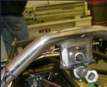
Wiring: front view
